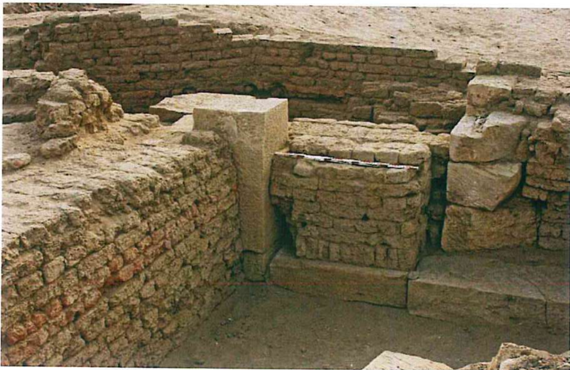
Fig. 5. Nağ' al-Hağar, late Roman fort. The south-east square corner tower T11 with a postern built of sandstone blocks, seen from the west, together with the later mud-brick walling, inserted when the entrance was blocked.
